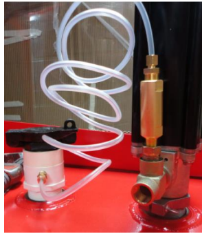
Figure 5 Pressure Relief Kit Installation
