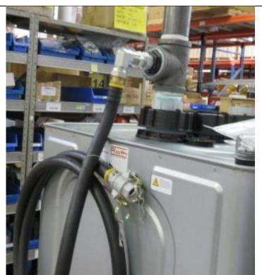
Make sure to attach the yellow coiled air hose to the <u>EXIT</u> <u>PORT ON THE ALARM</u> used on the waste tank.
